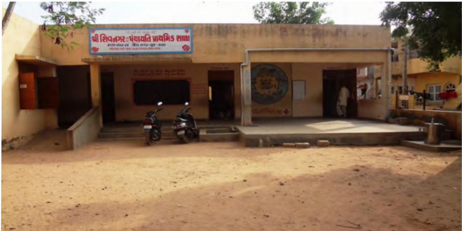
A groundwater recharge pit at Jubilee Colony (top) and an installed RRWH system in a government-run primary school at Shivnagar (bottom)
